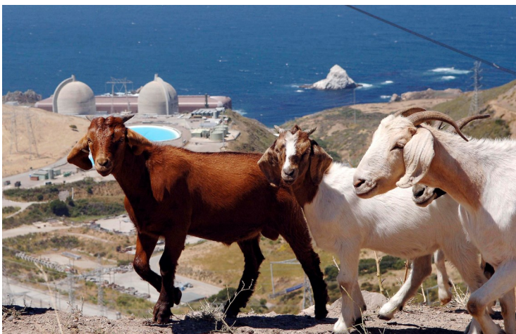
← A flock of goats walk on a hillside above Diablo Canyon nuclear power plant at Avila Beach, California in this June 22, 2005 REUTERS/Phil Klein//File Photo
